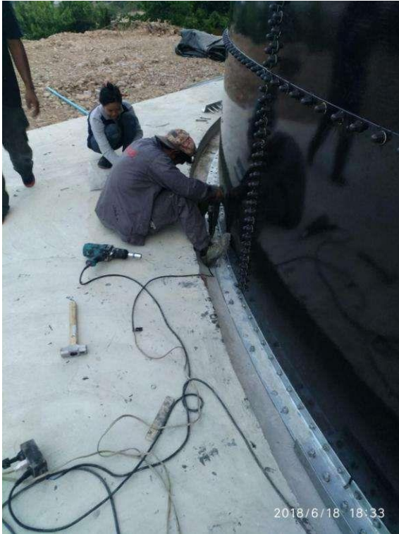
Install the base angles
