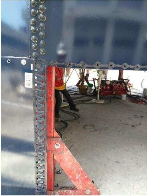
Apply the Sealant
